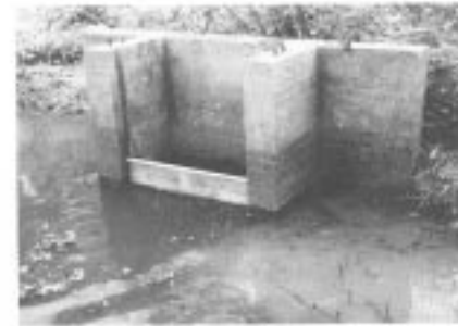
Figure 3. Water control structure
